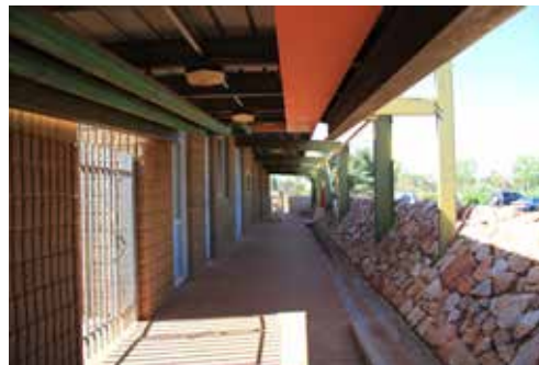
Deep verandahs around the external perimeter of the building provide protected circulation
