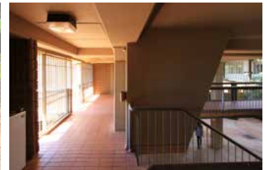
Heavy mass floors and walls of the perimeter buildings are protected from direct sun
