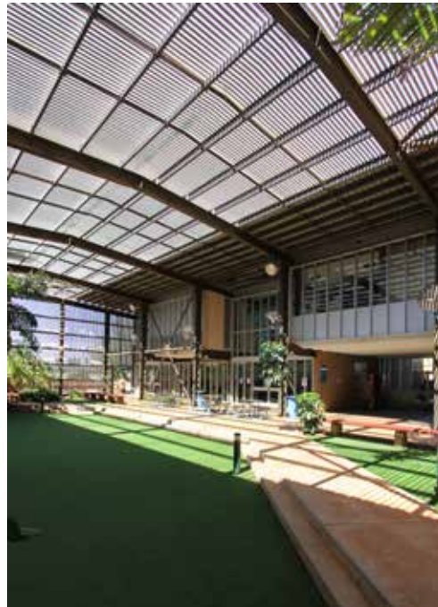
The central double volume courtyard with its permeable screen walls and roof protects classrooms and workshops from direct sun
